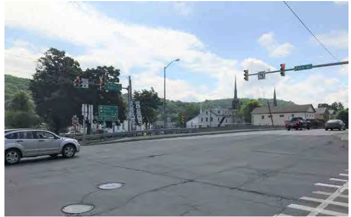
Existing north gateway at Park and Main St.
