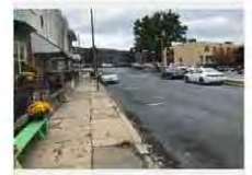
Sidewalk with uneven surfaces
