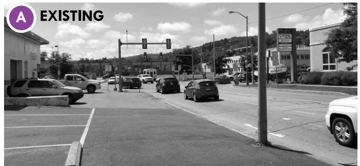
Existing South Gateway view from Main St.
