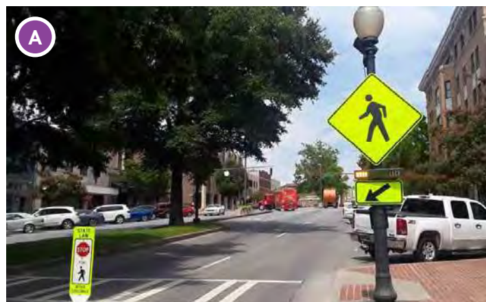
Image of flashing beacons to be installed along Main St.
