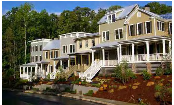
This image was a favorite option for the character of new townhomes that could be built on the edges of downtown Honesdale.
