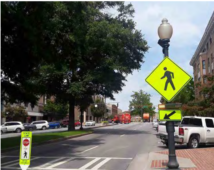
The photo above shows a street crossing with curb bump-outs and flashing beacons to keep pedestrians safe near busy traffic.
