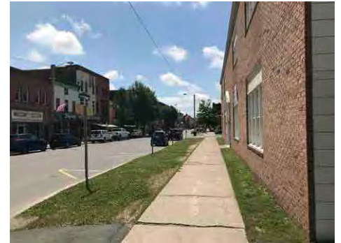
Existing small/cracked sidewalk along Main St.
