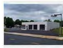
No landscaping along parking lot
