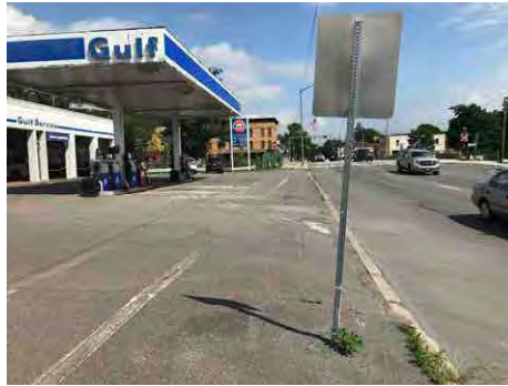
Existing asphalt sidewalk condition along Main St.
